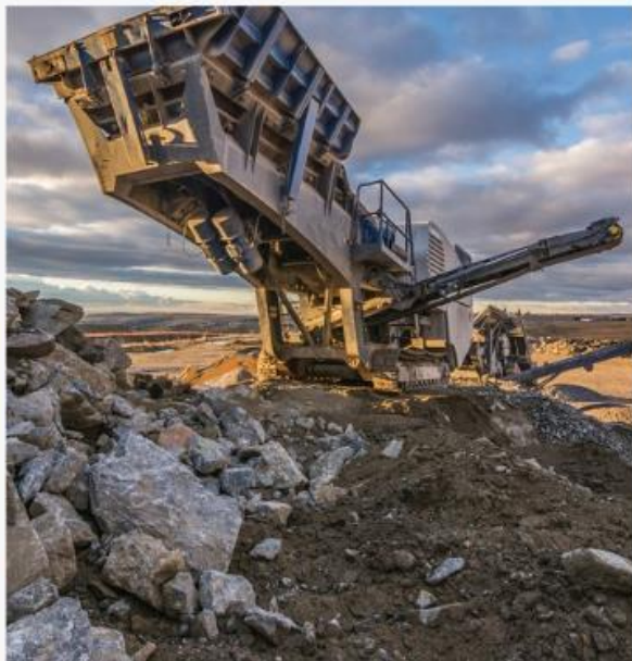
Construction: Rock Crusher
